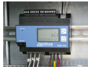
Power Analyzer • 20 kHz sampling rate • Memory limited (24 hours)
