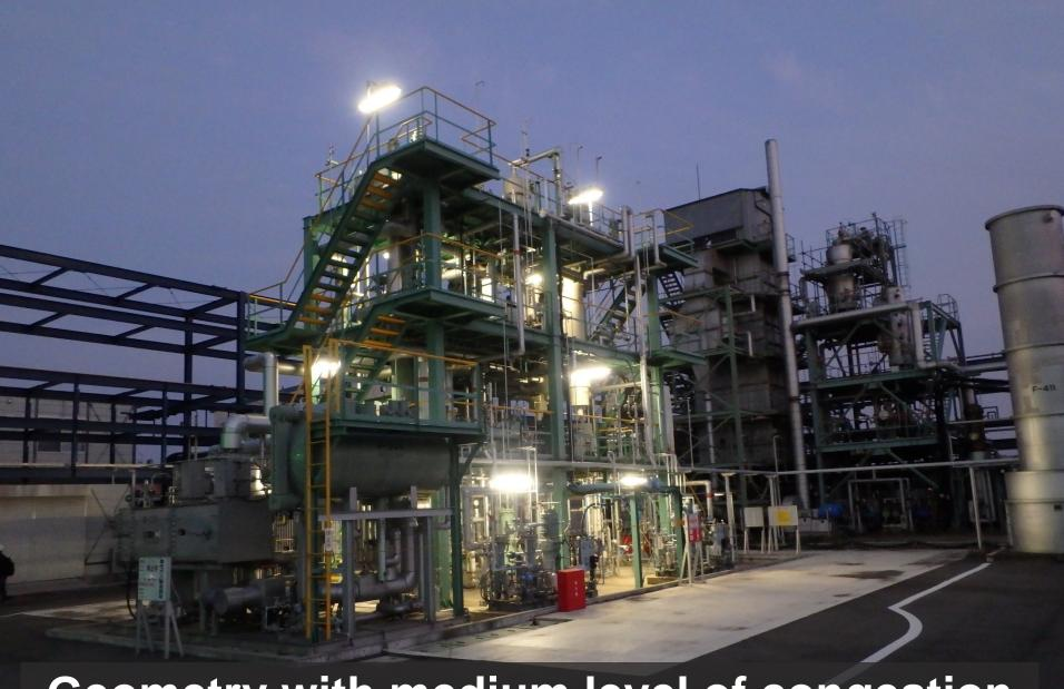
Geometry with medium level of congestion and low degree of confinement
