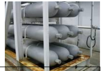
Cylinders at hydrogen station
